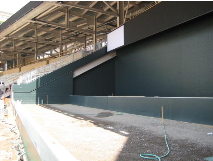
Photo 1 – Bullpen area soil placement
