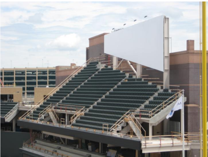
Photo 9 – Grandstand area seat installation
