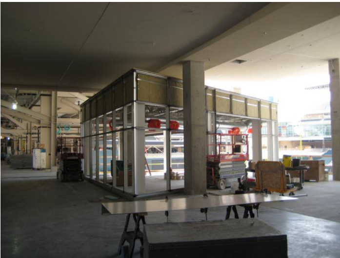
Photo 3 – Left field retail store framing
