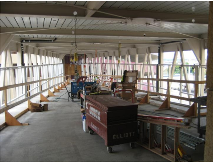
Photo 11 – Ramp A walkway connection
