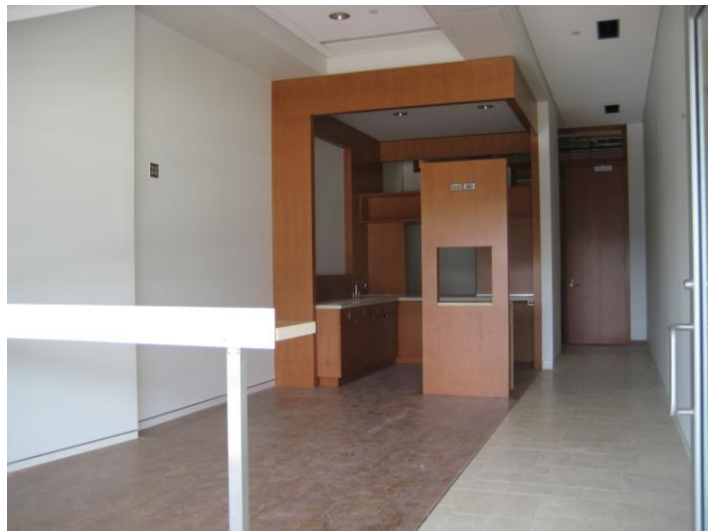
Photo 8 – Right field suites are nearing completion
