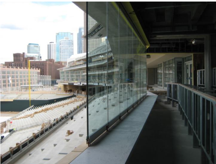
Photo 13 – Press Box glass installation
