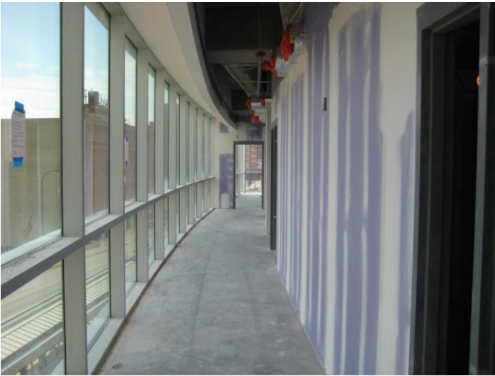
Photo 5 – Admin office walls are nearly ready for paint
