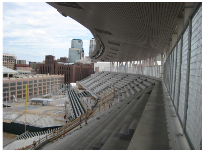
Photo 15 – Home Plate View seating area
